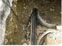
Depending on the situation, the fibre cable is pulled in from the cable manhole or handhole.
